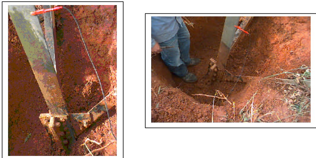
Fig.7 –Image of anodically polarized foundation
