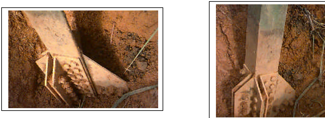
Fig.8 – Image of a cathodically polarized foundation
