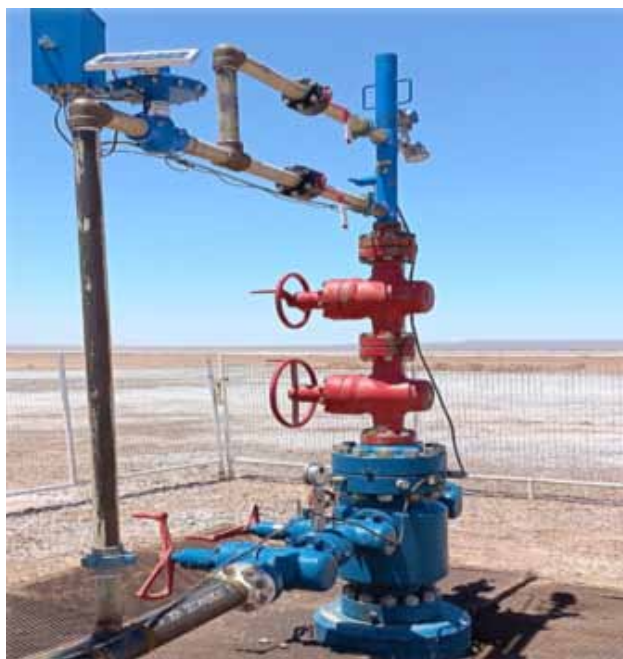
Figura 14. Plunger lift en shale oil de PAE.
