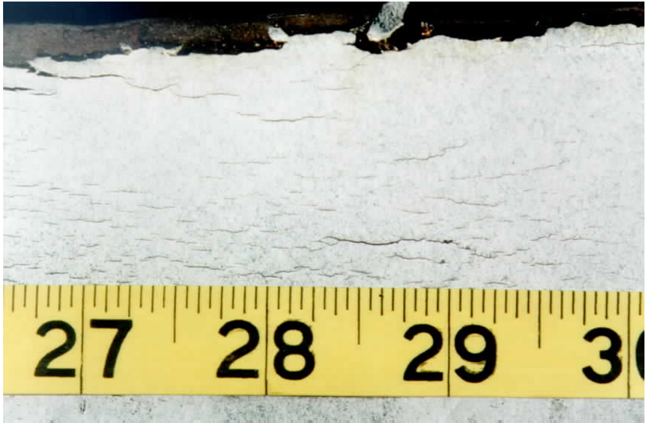
Figure 1. Optical photograph of near-neutral pH SCC colony following MPI inspection.
