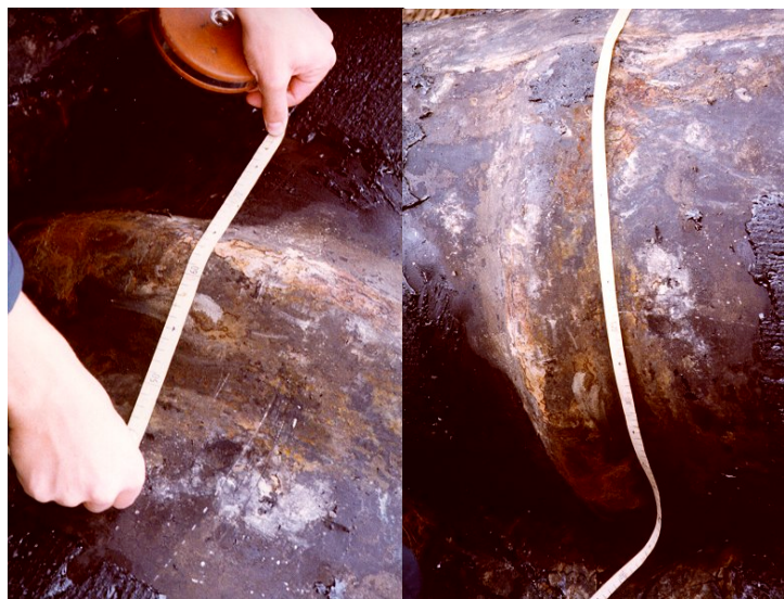
Fig 9 Verification of Wrinkle Dimensions in Cut-out Section
