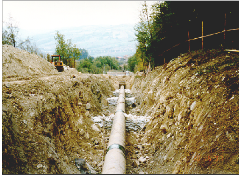
Fig 1 Pipeline Excavation for Stress Relief
