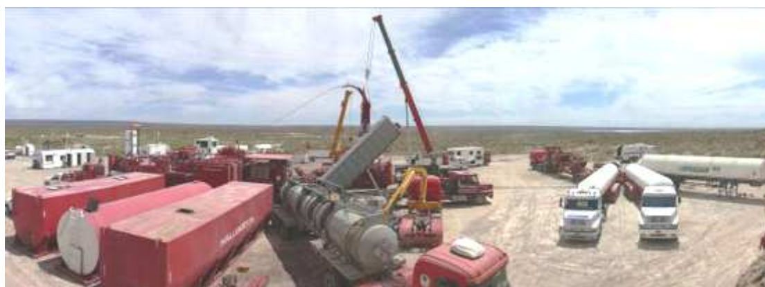
Fig. 8—Frac crew on location.
