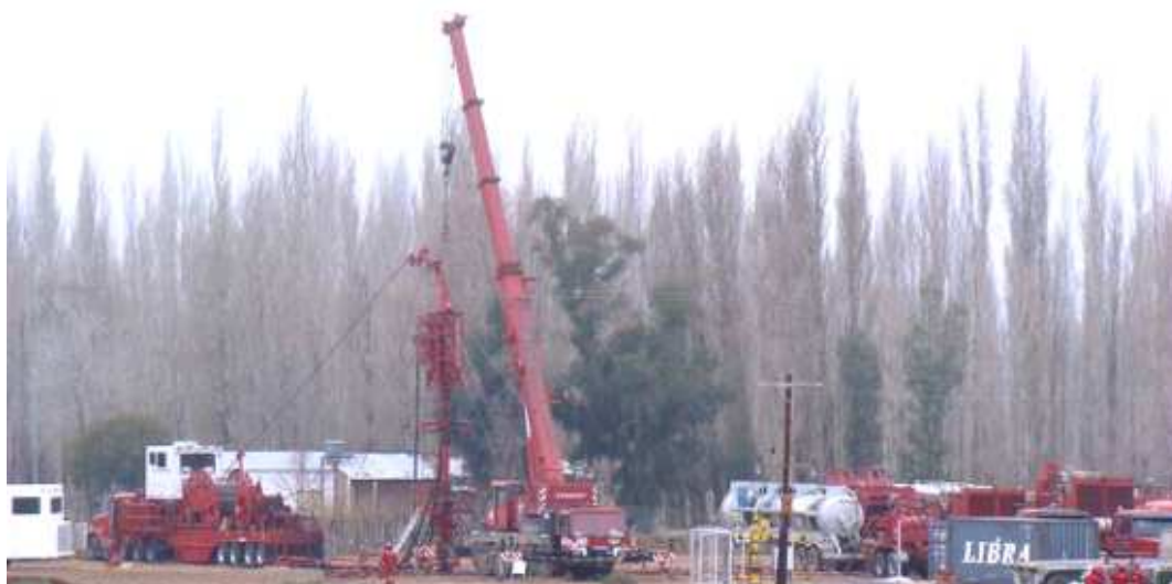
Fig. 11—Frac Crew on location.
