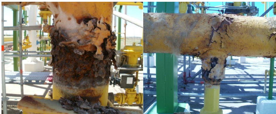
Figura 18: Zonas susceptibles a CUI II – Planta Solar
