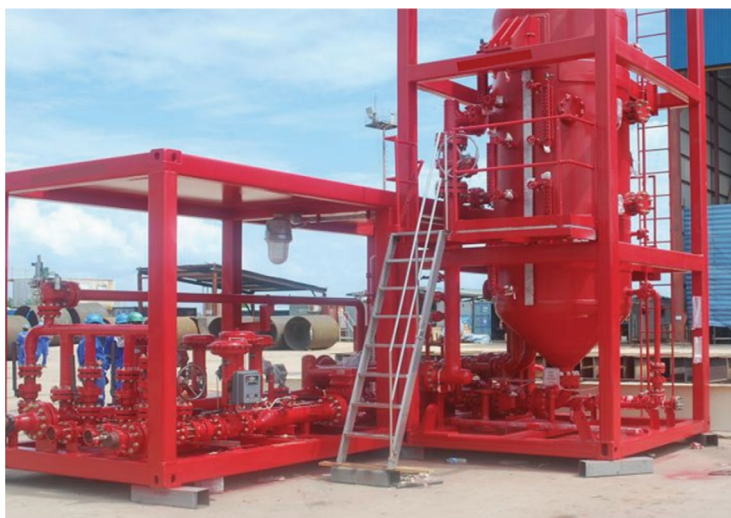
Figure 1. 4-phase separator and control skid
