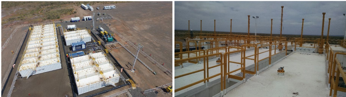
Figure 12. Tanks runways and railings
