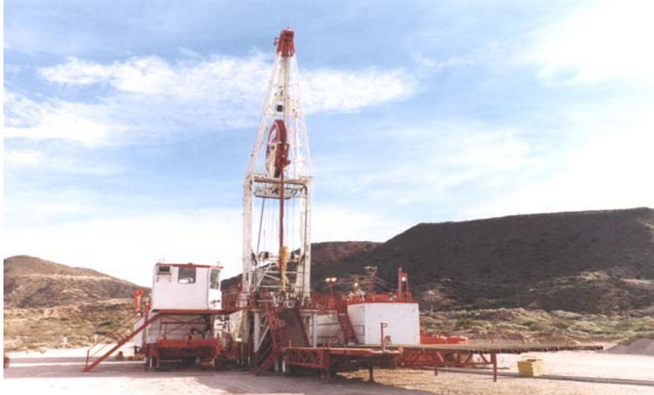
UNIDAD DE COILED TUBING DRILLING
