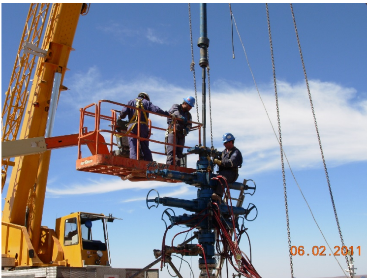
Fig. 10 Operators installing BHA using Double BOP (double safety barriers) and Extra Clamp and safety platform
