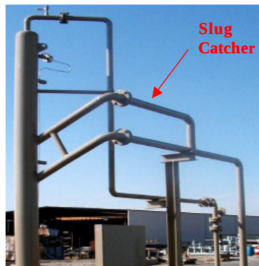
Figure 5. Slug catcher on a GLCC system
