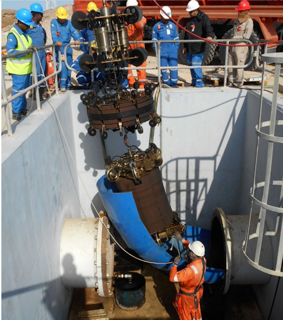
Figure 5 Installing a robotic UTWM tool using a slide into a spool-piece's removed entry point.
